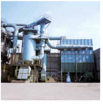
We select the appropriate dust collection equipment for each application after careful consideration. An example is the facility of changing over to a dry-type filter if no explosions are expected in the shredder. This filter provides an even better exhaust air quality than our wet scrubber.
