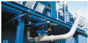
When ducts carrying material pass through fire protection barriers, safety elements, such as quick-closing firegates or fire protection dampers, can be used to isolate individual fire sections from one another.
