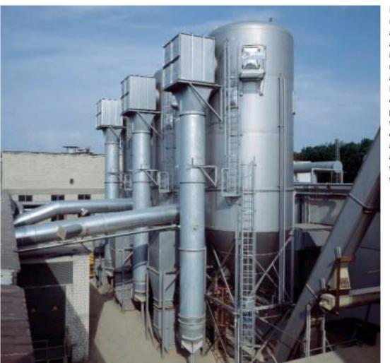
Pressure-shock-resistant round bag filter plants with amply sized explosion vents are used in the chipboard industry for surface sanding machines where a large amount of dust is produced. Ducts and pipework with explosion vents prevent the pressure wave from being transferred to downstream equipment. Should, however, a dust explosion occur despite all the safety measures taken, the explosion vents minimise the damage and downtime.
