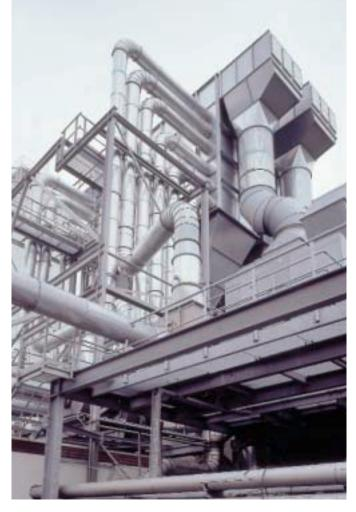
Amply sized explosion vents in the return air ducts and an 180 degree bend prevent the pressure wave being propagated in the workshop.
