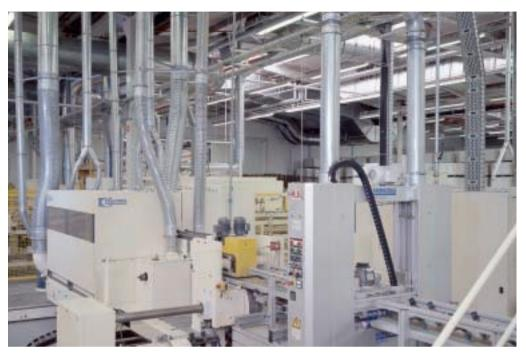
Venti plants can deal with over 100 suction points. Collected dust and chips are carried to the filter system and the following heat recovery plant via a main duct. Air volumes of over 300,000 m<sup>3</sup>/h can be exchanged in this way.
