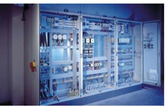
Of particular importance in a safety concept is the local monitoring equipment, such as, for example, infrared detectors, spark recognition plants, pressure monitors and level detectors. Evaluation of the signals received and the measures which must be taken accordingly is carried out by the controls, designed by Venti Oelde.
